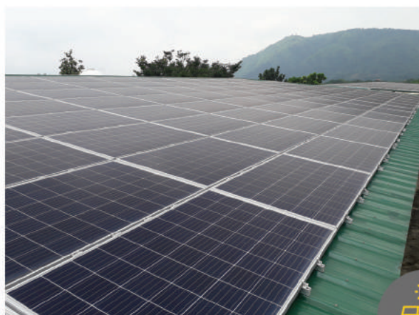
The 99.9 kWp Own-Use Rooftop Solar Photovoltaic (PV) System in FEU- Roosevelt in Rizal
