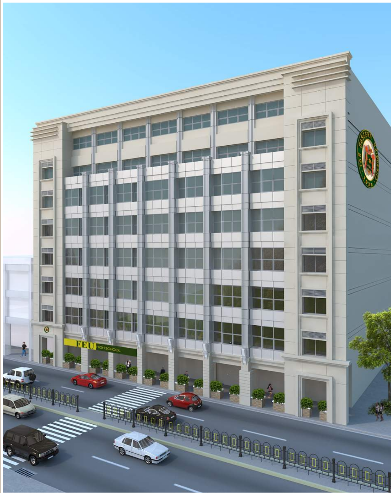
Far Eastern University High School Building Facade Nicanor Reyes Street, Sampaloc, Manila
